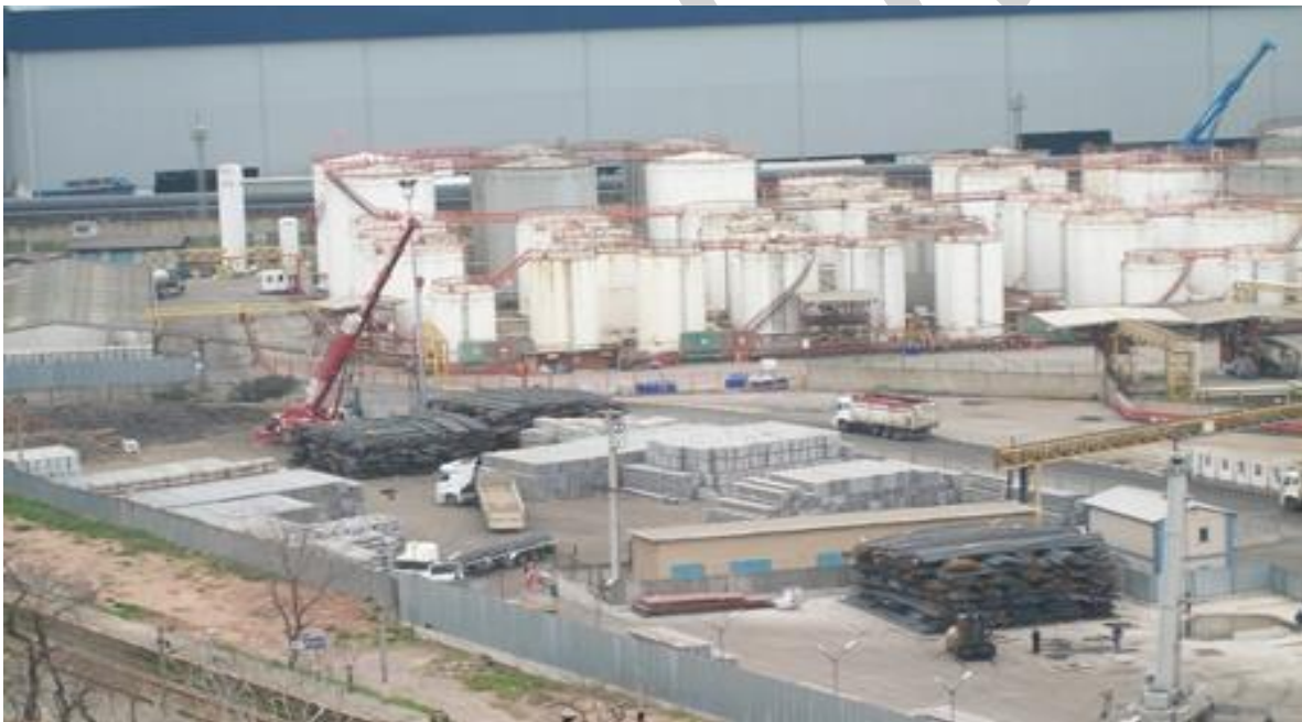
Figure 1.2 External View of Facility 2
