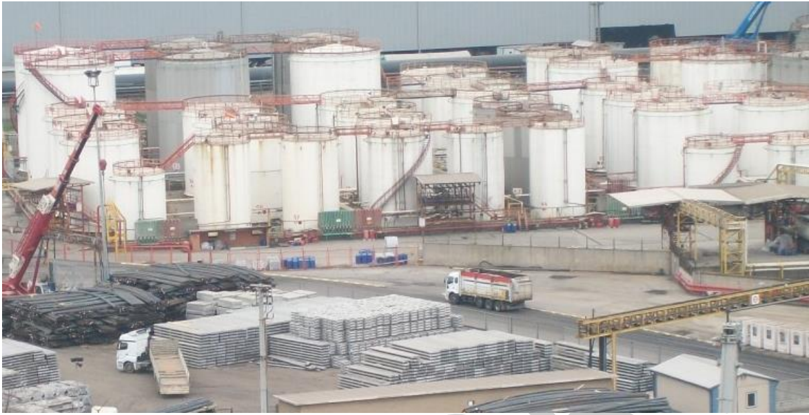
Figure 1.1 External View of Facility 1
