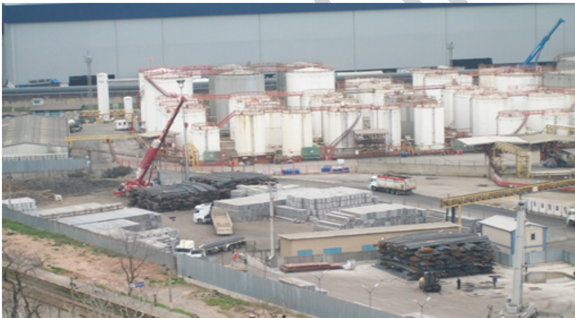
Figure 1.2 External View of Facility 2
