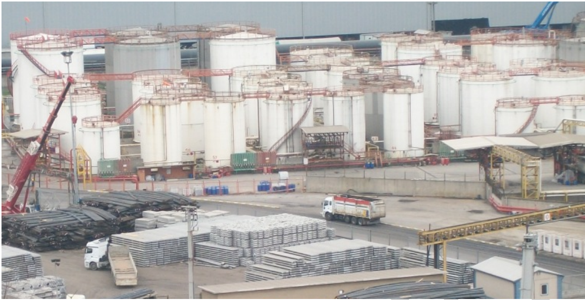
Figure 1.1 External View of Facility 1
