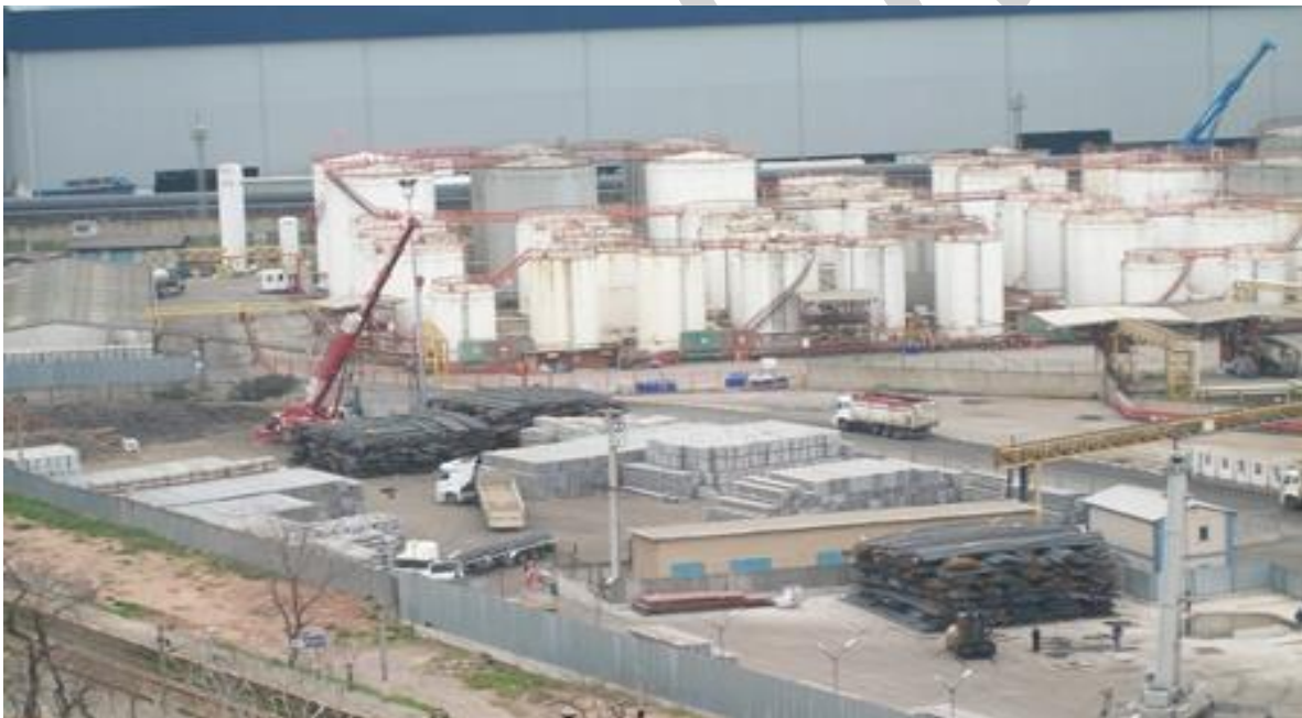
Figure 1.2 External View of Facility 2
